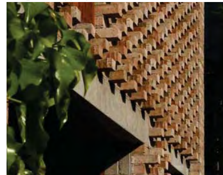
fig. 9.5 Masonry Bond Texture
