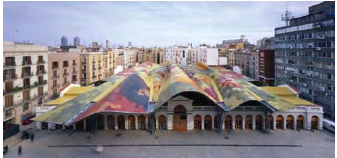
fig. 6.30 View of Roof
