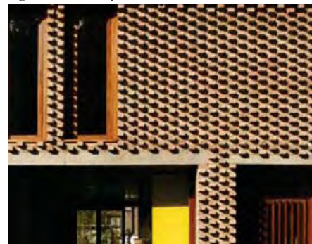
fig. 9.9 Masonry Bond Texture
