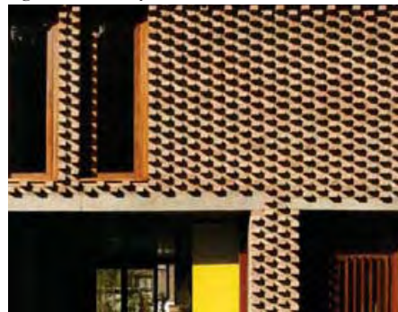
fig. 9.9 Masonry Bond Texture
