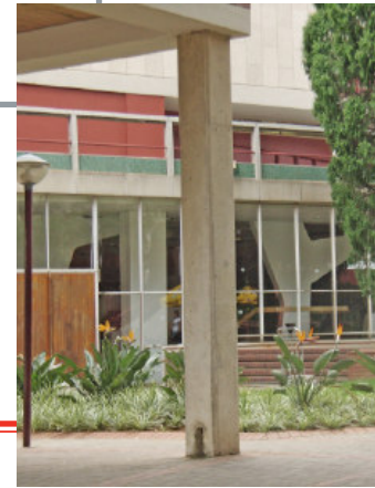
off-shutter reinforced concrete
