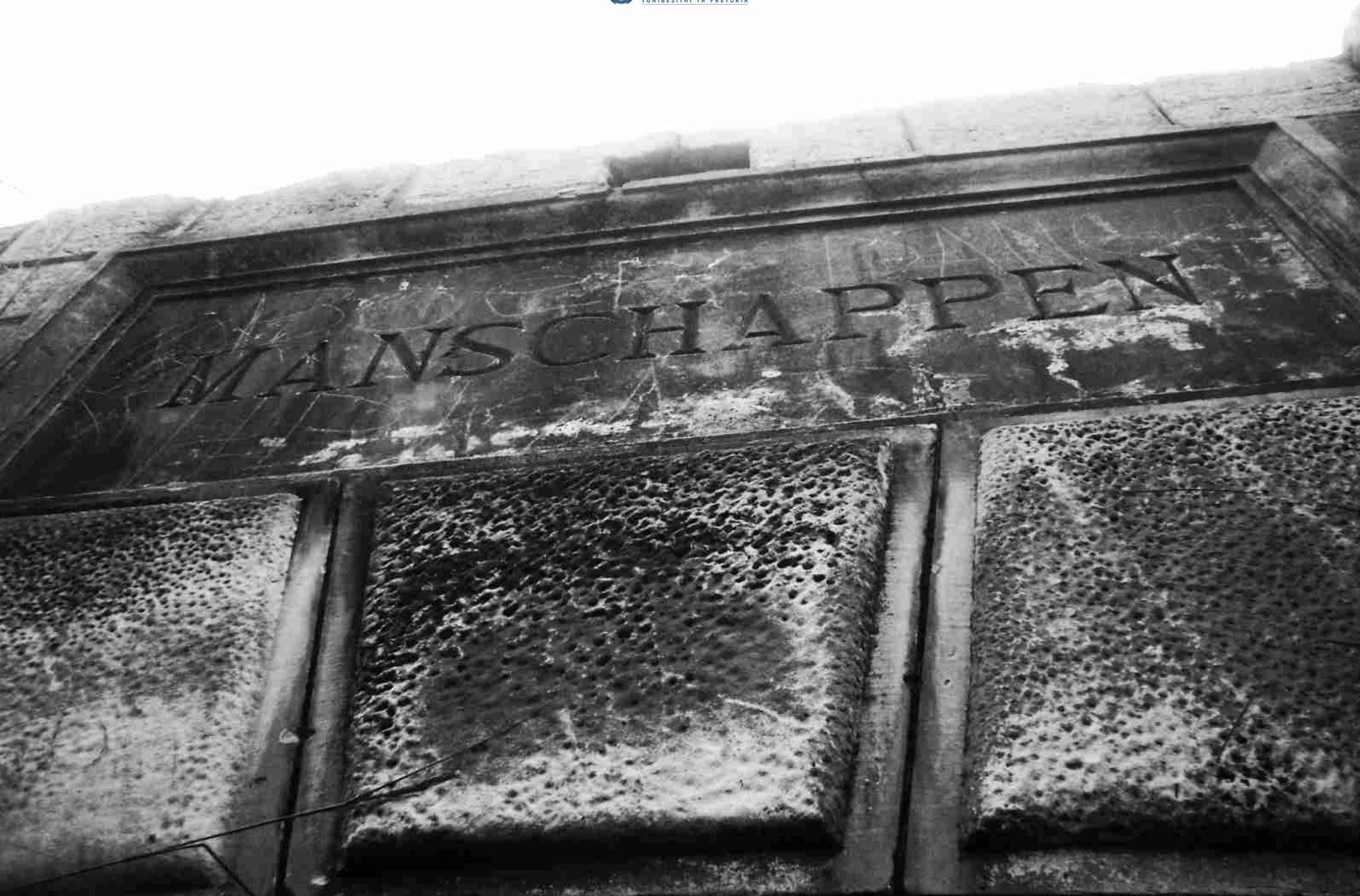
Fig. 2.37. Photo of the Manschappen provisions room. (2010)
