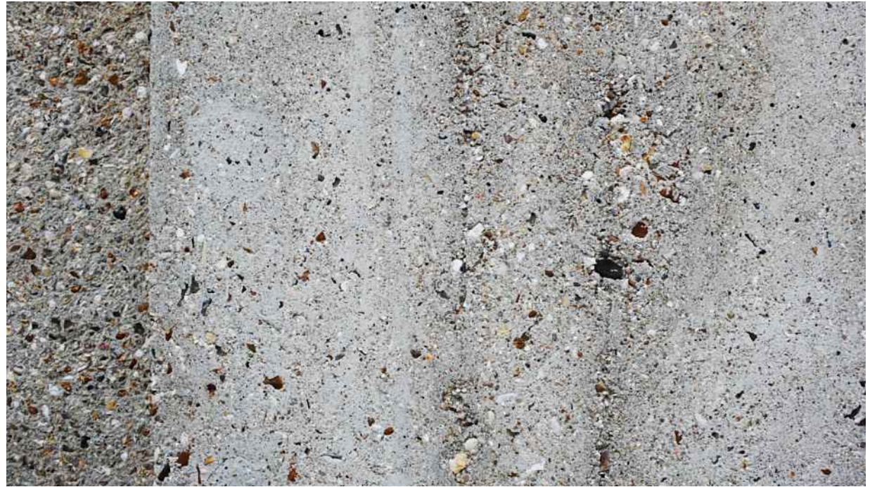
fig. 6.10. The Beton Brüt finish the author intends using. (2010)
