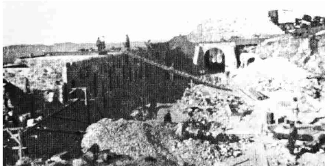
Fig. 2.26. Fort Daspoortrand during construction. (1998: 59)
