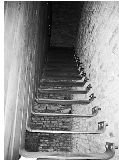
fig. 6.6 - 6.8. Scarpa's steel stair connection detail. (centralbranchlibrary.com:2010)
