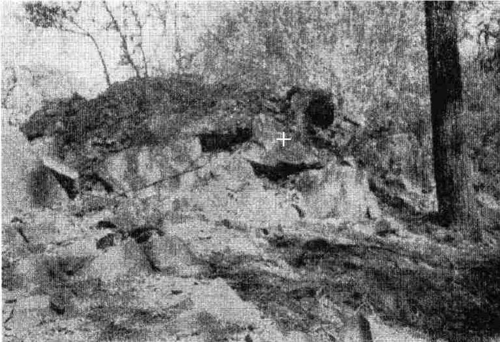
Fig. 2.19. Remains of the Klapperkop Blockhouse. (1998: 91)
