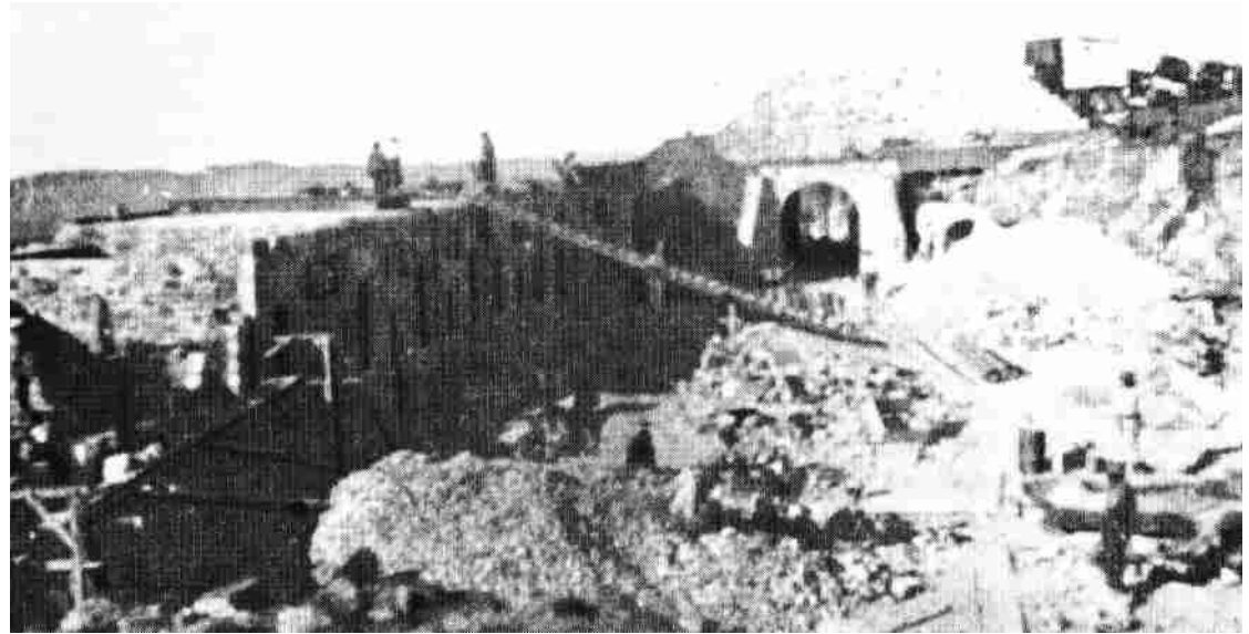
Fig. 2.26. Fort Daspoortrand during construction. (1998: 59)
