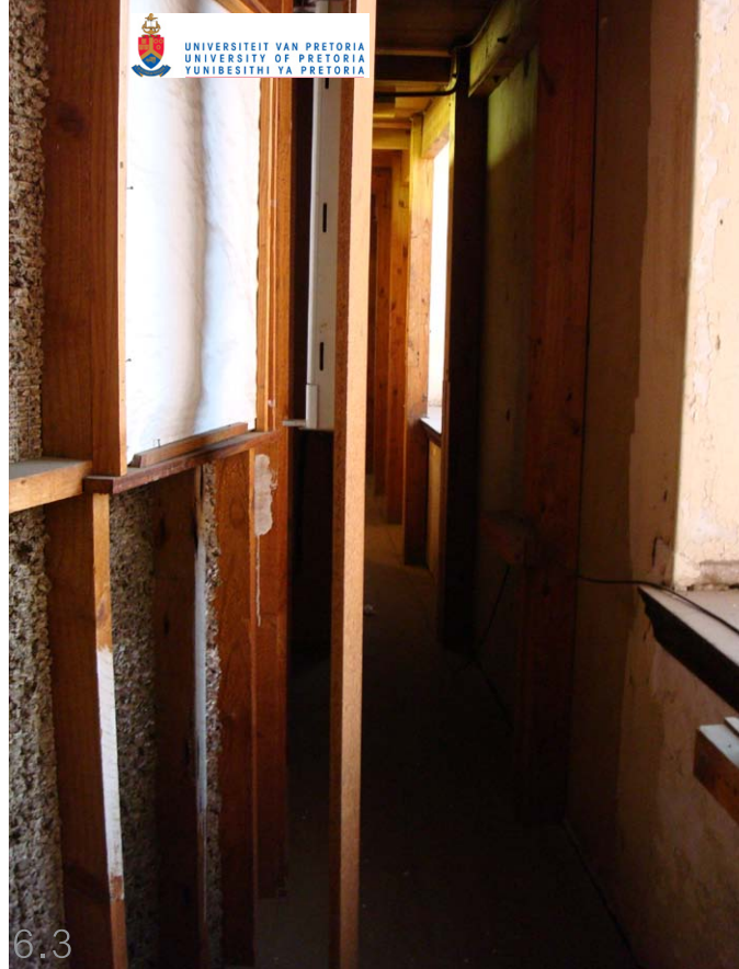
Figure 6.3: Exhibition panels blocking natural light from entering the hall
