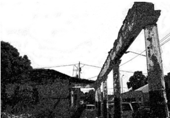
Figure 5.1 Partly demolished structure in Grand Street (Author, 2010).
