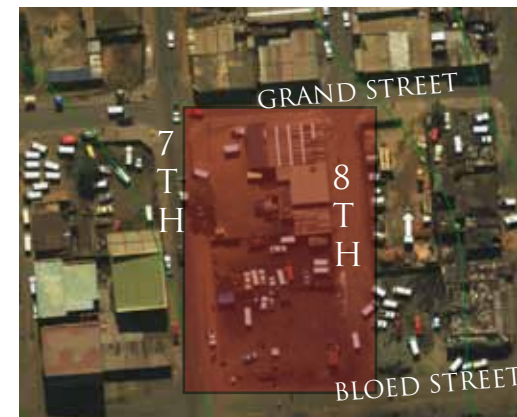
Figure 5.3 Selected Site. Previous structures have been demolished and the site is mostly open (Munitoria, 2010)
