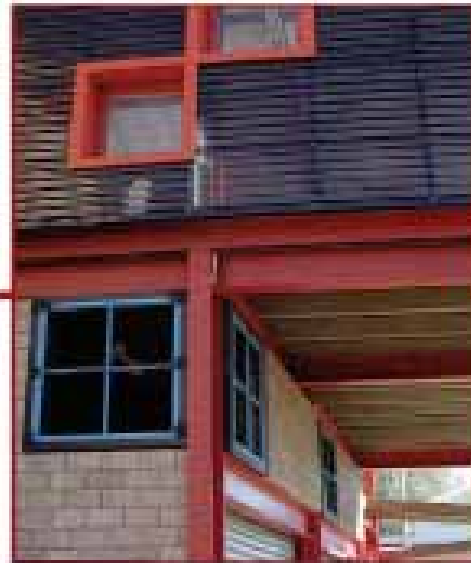
Figure 4.2 Polycarbonate sheeting, steel frame and brickwork (Decklar et al., 2008 : 48-49).
