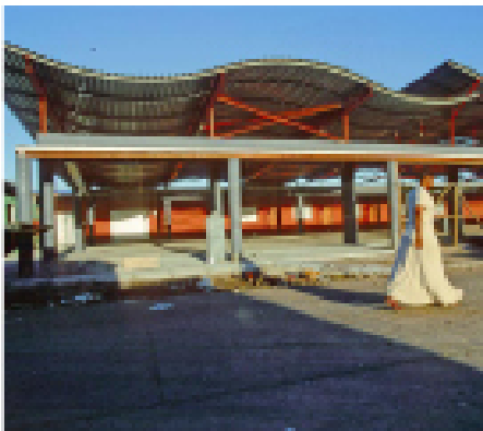
Figure 4.12 Roof over market space with shops at the back. Clear distinction between spaces and programme (Smuts, 1999 : 44).
