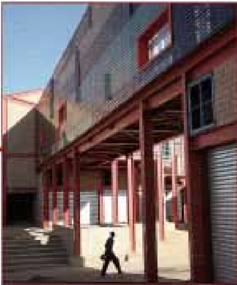
Figure 4.1 Bridge connecting two corners of site (Decklar et al., 2008 : 48-49).
