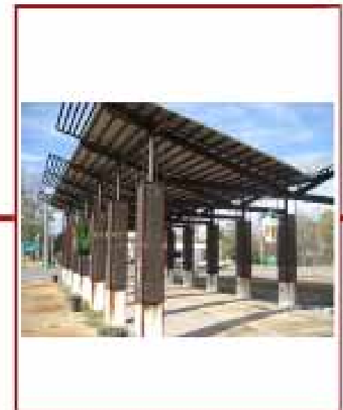
Figure 4.19 Construction of columns with concrete, steel and steel mesh to create bulky appearance more economic than column made of only concrete (Oppenheimer, 2002:134).
