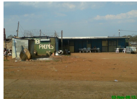
Figure 2.5 Trading structures on Hans Strijdom Road
