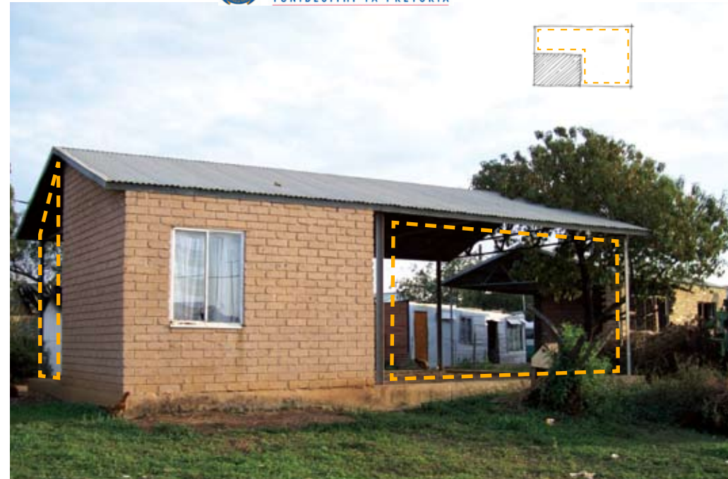
Fig. 14 Government subsidised house requiring owner to fund any new additions, Mamelodi, 2008.
