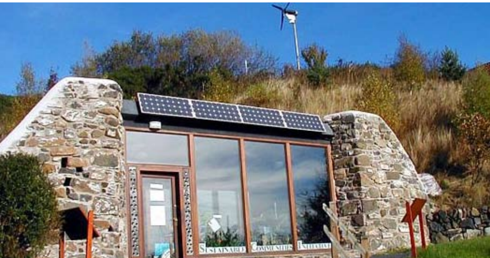
Fig. 12 The Earthship, built mainly from recycled materials, the sustainability centre uses renewable energy and water recycling strategies to increase its self-efficiency.
