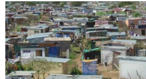
Fig. 22 Lusaka informal settlement, Pretoria, South Africa
