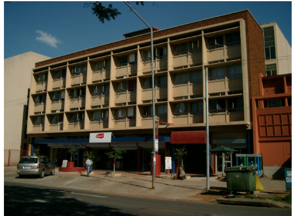
Illustration 5.3: The inconspicuous facade of the TAU building with shops opening up onto the street
