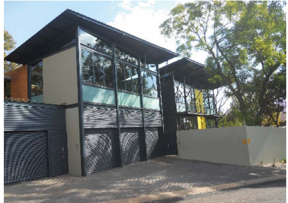
Figure 5.33: View of the street elevation
