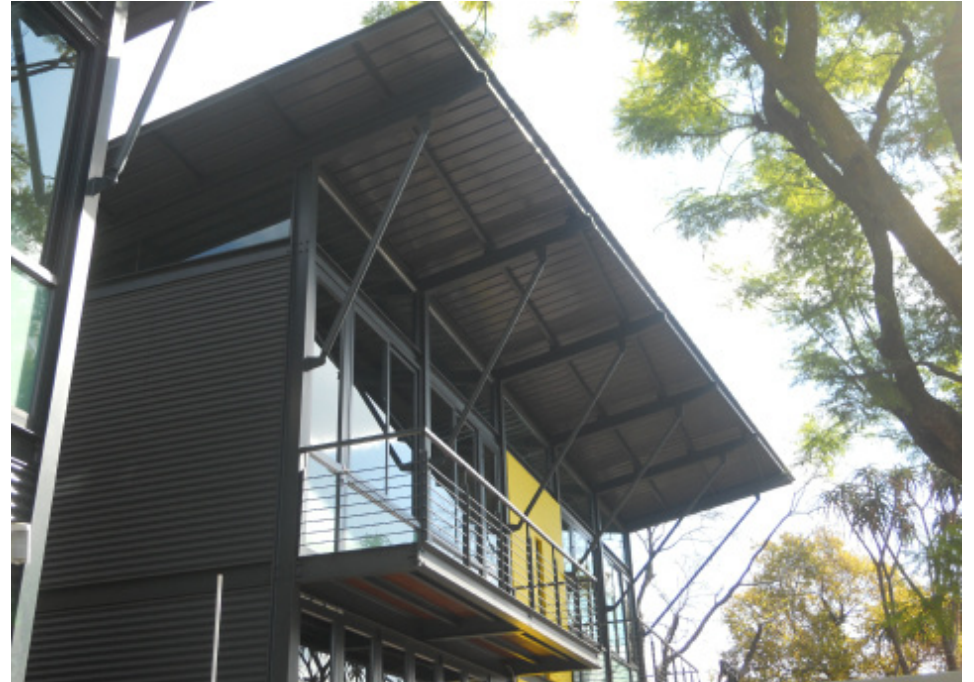
Clockwise from top right Figure 5.35: View of the various skin construction materials Figure 5.36: View of the balcony from the street showing the roof structure Figure 5.37: View during construction showing the structural frame and infill
