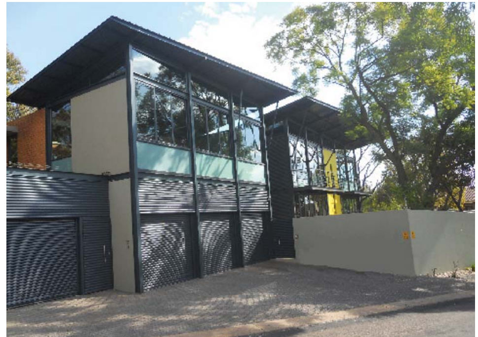
Figure 5.33: View of the street elevation
