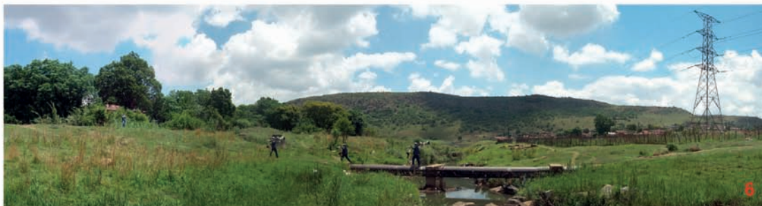
Figure 99: Old sewer pipe used as a bridge'
