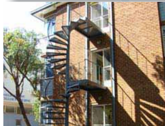
Spiral staircase at Marketing building
