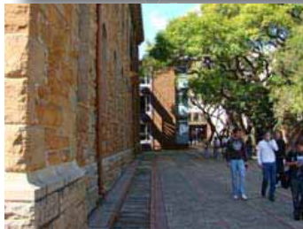
Southern stone edge of Old Arts building
