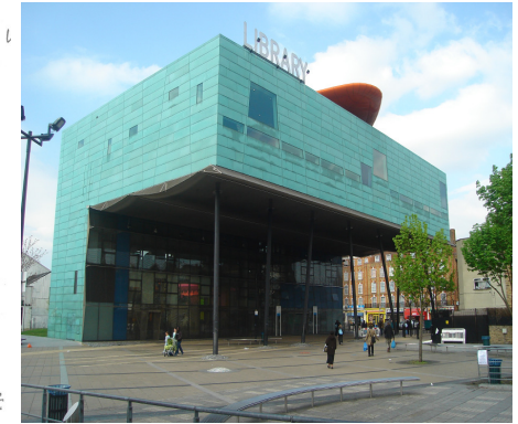
illus. 5.7b Exterior of Peckham Library
