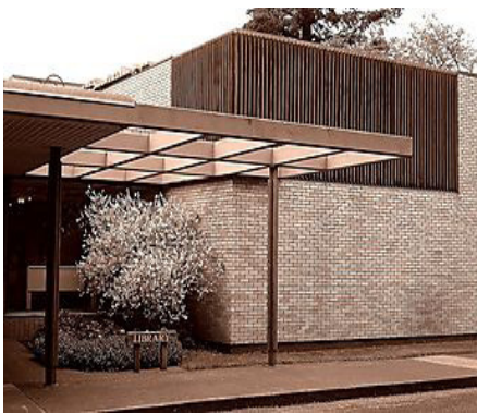
illus. 5.6a Brick exterior
