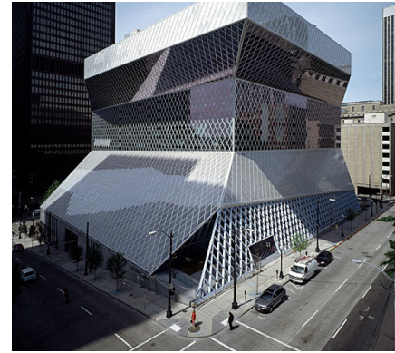
illus. 5.22a Exterior view of Seattle Central Library
