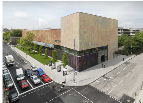
illus. 5.15b Photo of corner with entrance away from corner
