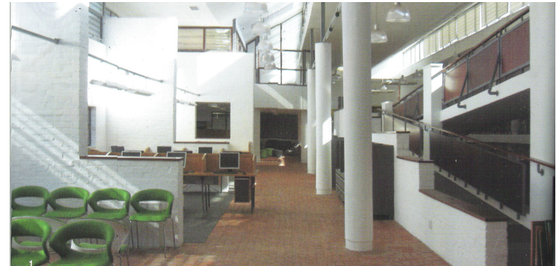
illus. 5.17 Main circulation space with brick paving, and natural lighting from saw-tooth roof clere storey windows
