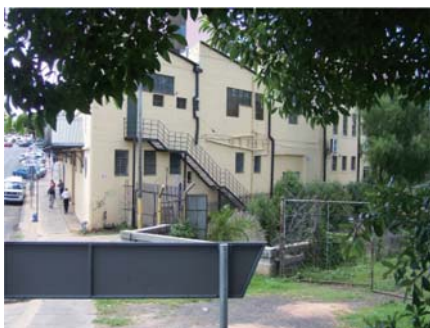
Figure 7.5.21. Building adjacent to Walkerspruit (Author,2011). The building in the background fronts Pretorius street and the western facade fronts onto Walkerspruit and Caledonian. The building is currently occupied by a church and Christian book store.
