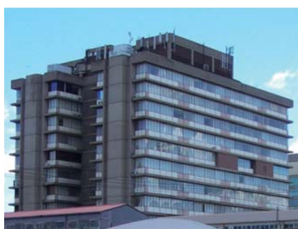
Figure 7.5.25. Kingsley Centre viewed from the south east on Pretorius Street (Author,2011). The building is the tallest building in the block. Is also offices for the department of Arts and Culture for Pretoria.
