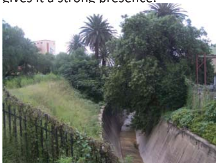
Figure 7.5.13. View of Walkerspruit running northwards along the western edge of the site (Author,2011). To the left is a wedge of closed off green space between the Apies river and Walkerspruit, could become a possible open space link to the site.
