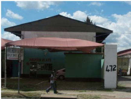
Figure B. 37 & Figure B. 38 B - stand 1083 (Author, 2011). Description : Double storey main workshop and reception User : Arcadia glass and frame work (automotive) Analysis : Valuable concrete frame building, part of series of longitudinal warehouse structures Intervention : activate buildings along street facade, possible mixed use work live units/ double volume retail spaces
