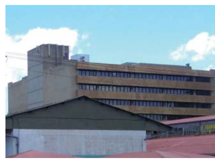
Figure 7.5.26. Benstra building (Author,2011). The south and western facades of this multi storey building defines the project site. The buildings northern facade create a strong urban edge onto church street but offers no pedestrian interface with the street.
