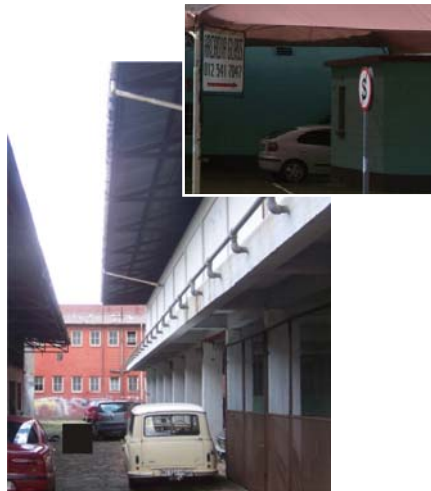
Figure B. 39 & Figure B. 40 G - stand 1183 (Author, 2011). Description : Covered parking and outbuildings User : Arcadia glass and frame work (automotive) Analysis : no interface between street and pedestrians Intervention : removal of canopy structure, space between building to form part of access into precinct
