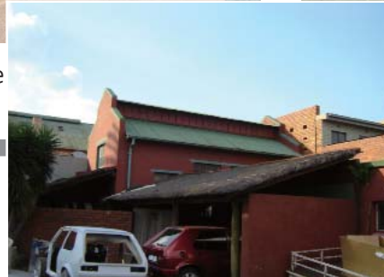
Figure 7.3.14 Photo of character of the existing building to be retained (Author, 2011).
