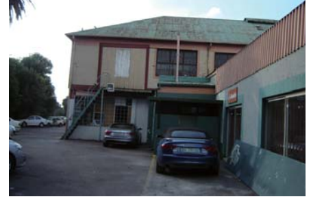
Figure B. 11 & Figure B. 12 A - stand 1053 (Author, 2011). Description : Double storey workshop User : Automotive Analysis : Heritage building, contributes to character of the precinct. Building defines and lends scale to proposed open spaces. Intervention : re-use arts and craft workshops/Restaurant/ exhibition, arts performance space and photography.
