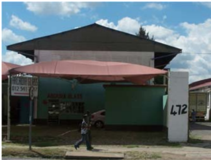
Figure B. 37 & Figure B. 38 B - stand 1083 (Author, 2011). Description : Double storey main workshop and reception User : Arcadia glass and frame work (automotive) Analysis : Valuable concrete frame building, part of series of longitudinal warehouse structures Intervention : activate buildings along street facade, possible mixed use work live units/ double volume retail spaces
