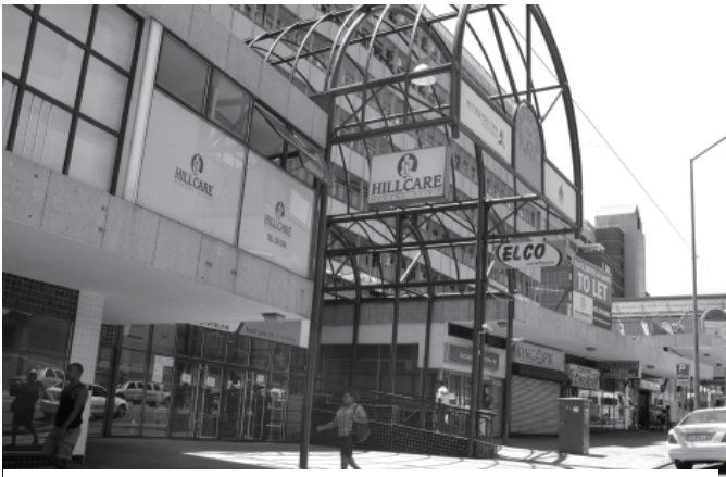
Figure A. 13. Photo of the character of commercial buildings opposite the site (Author, 2011).
