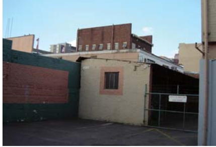
Figure B. 9 & Figure B. 10 D - 1053 (Author, 2011). Description : Covered parking. User : Automotive Analysis : Footprint important within structures. Structure is Neutral towards proposed development. Intervention : removal to increase access to proposed precinct open square.
