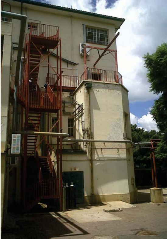
Illustration 3.3 The degeneration of the Tshwane District Hospital
