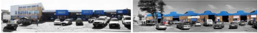
Fig 6.39: Fitting centres in Zeller Street, Pretoria West, Photos by Author 2011
