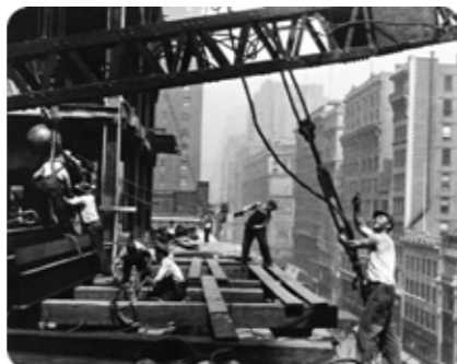
Fig 2.18: 1931 Construction of The Empire State Building (Acid Cow 2010)
