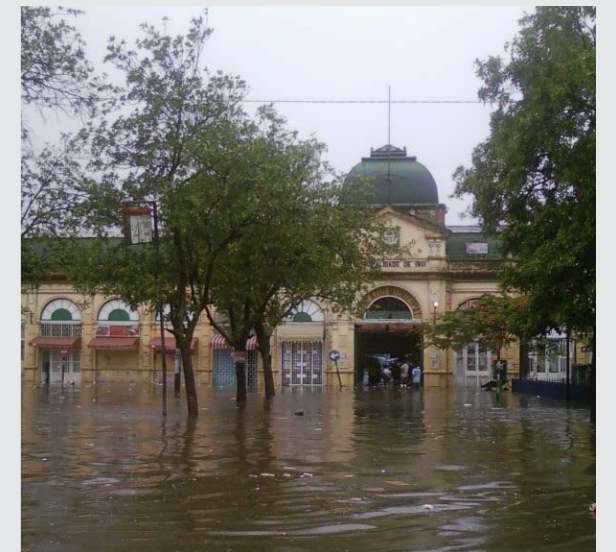
Illus. 88: Flooding, Ave 25 de Setembro, in front of Maputo Central Market
