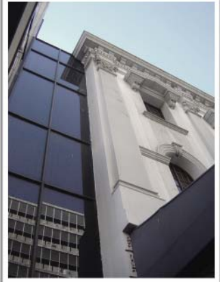
2.11 OPERA PLAZA. RESTORATION
