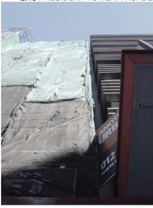
2.18 PRESIDENT TOWER. FACADE
