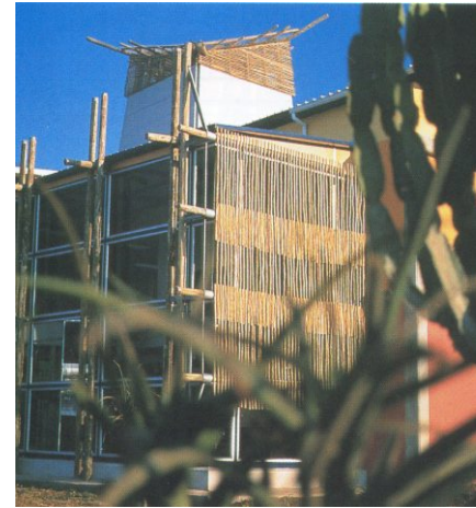
4.6 Corner detail. Natural materials used give the building a unique regional quality.
