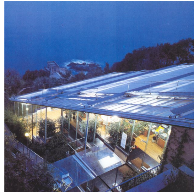
4.1 During the day, the building disappears into the slope, while at night it seems to step away from the slope, completely exposing the interior as its own environment.
