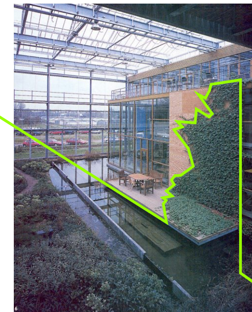
4.9 Internal garden. The building within a building concept creates a giant air-gap between the interior and exterior that provides maximum temperature control. This allows for the use of large expanses of glass that seems to draw the external environment indoors.
