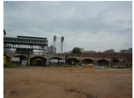
Figure. 99. View of Nelson Mandela Bridge
