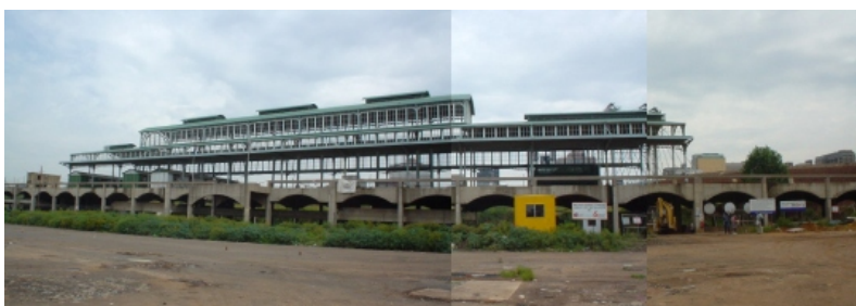
Figure 21. Old Parktown Station
