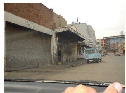
Figure 20. Derelict buildings in the vicinity
