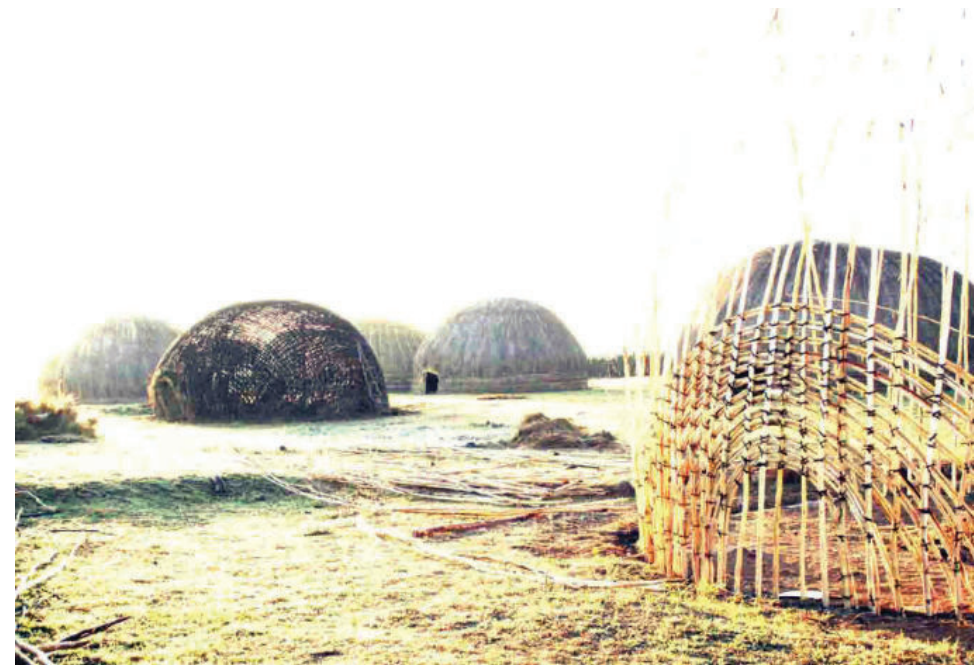
(b) Zulu huts in various stages of construction Author, 2010
