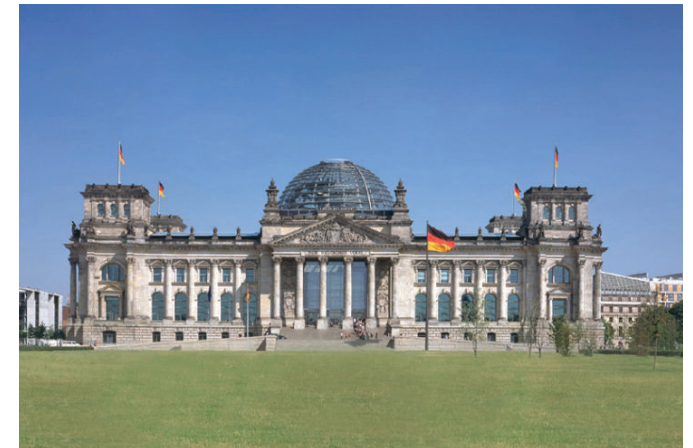
Figure 4.17: View of the Renovated Building as a Contemporary Icon ( http://www.fosterandpartners.com )
