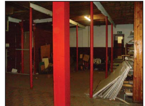
fig.6.14. Steel supports inserted for wooden flooring above
