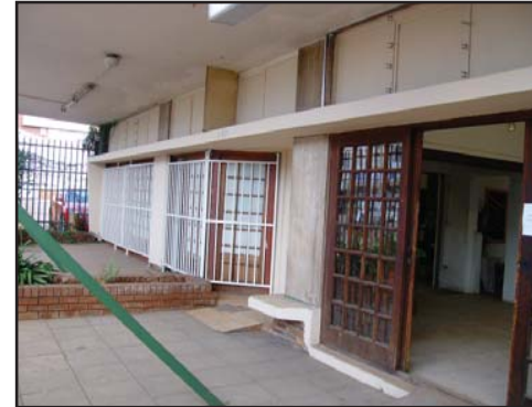
fig.6.10. Main pedestrian entrance (previously shop fronts)
