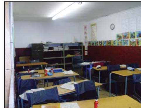
fig.6.12. Drywall partitioning is used to sub-divide the warehouse into classroom spaces (minimum natural lighting and ventilation)
