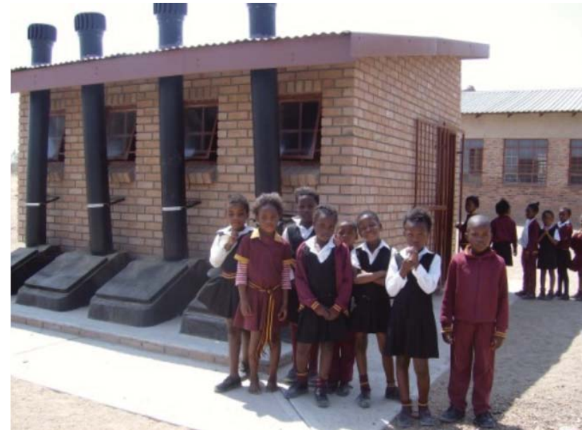
Fig.171.(Enviro-Options) View of installed enviro-loos
