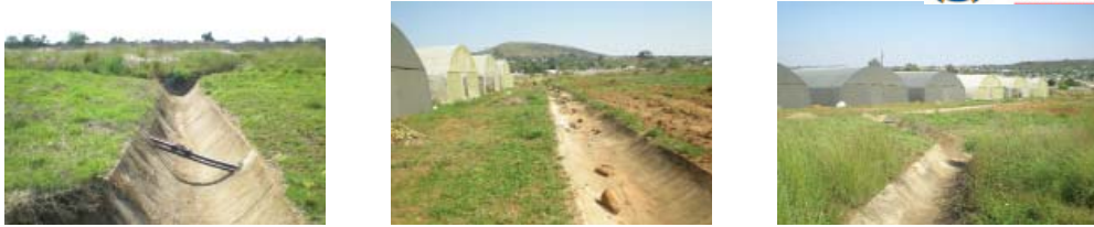
Fig.64.(By Author) Views of existing canal
