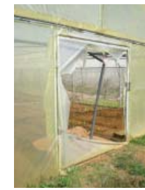
Fig.60.(By Author) View of an agricultural tunnel showing disrepair
