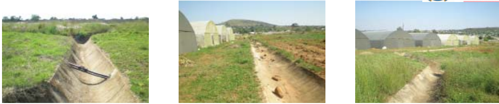
Fig.64.(By Author) Views of existing canal
