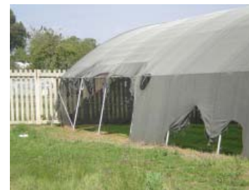
Fig.59.(By Author) View of an agricultural tunnel showing disrepair
