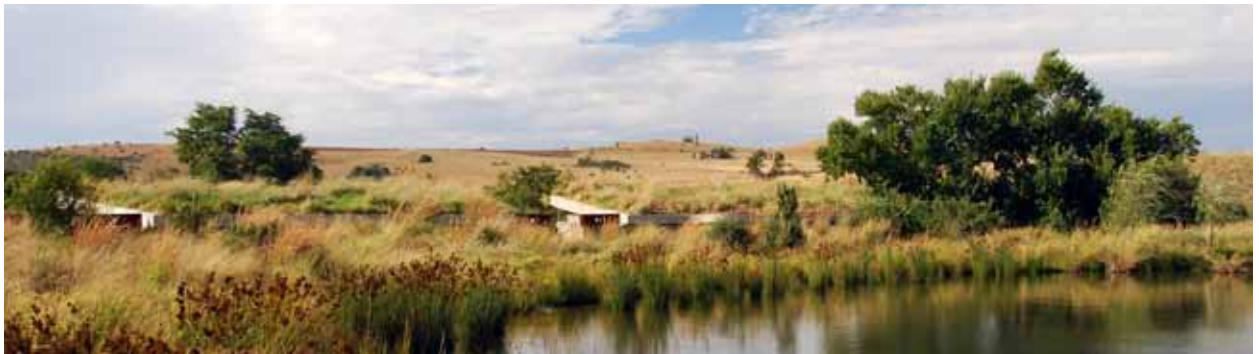
Figure 4.10 View over the planted sod roofs
