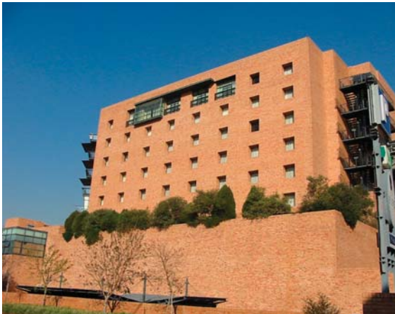
Figure 4 -1 Exterior of Hyatt Hotel, Jhb.
