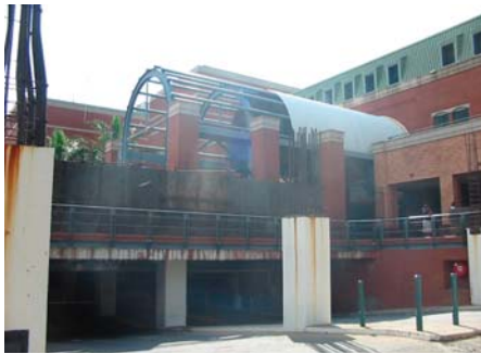
Figure 9 -1 Entrance/ Exit ramp from basement
