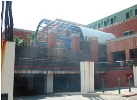
Figure 9 -1 Entrance/ Exit ramp from basement
