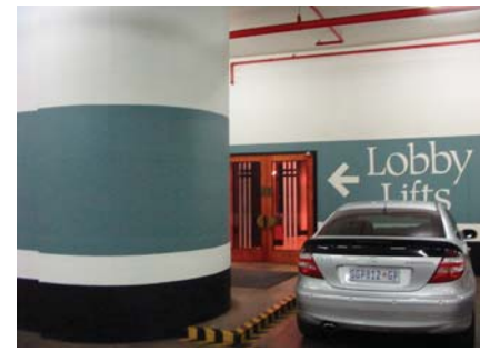
Figure 4 -10 Basement Exit, to hotel reception
