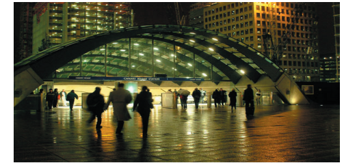
FIG 017 Glass and steel canopy entrance
