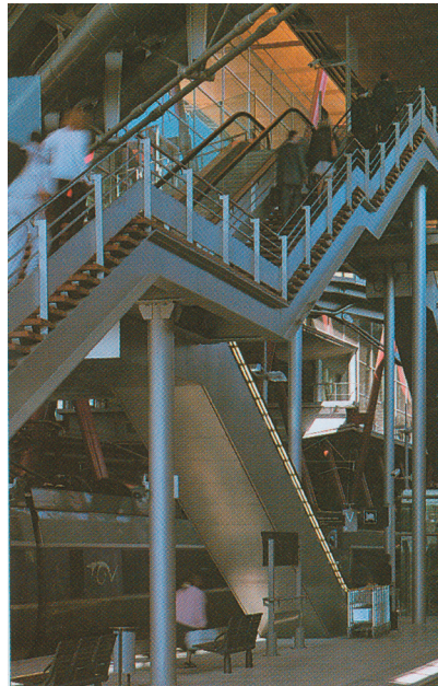
FIG 019 Staircase at Valence station expressing passenger routes
