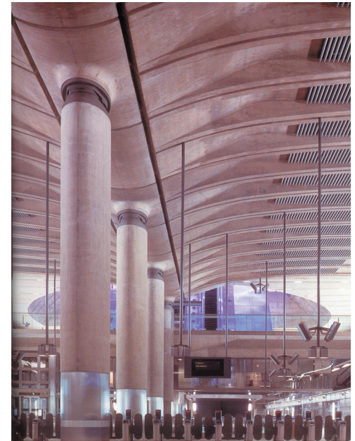
FIG 018 Open concrete concourse with ticketing machines
