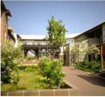
Figure 6.43: Low rise community buildings
