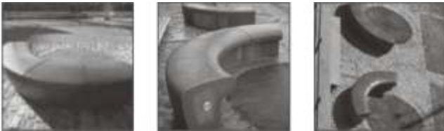
Figure 4.25-27: CARNAMUSA: Alejandra Ferrugia & Daniel D'Andrea. Fore pressed pieces shaped like bits linked one to the other by a galvanized iron rod.
