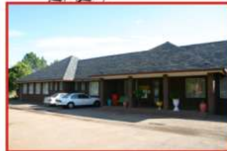
Figure 6.34: Family and child care unit The facility houses children on the campus and also functions as the information desk for the hospital. The accommodation of both functions, in a single building, is not ideal.
