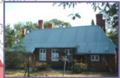
Figure 6.32: Historic house The house is currently occupied by staff members, but the proposal is for it to serve as a museum for the hospital and tea garden in the gateway precinct. The concept is to preserve the historic context and create a point of interest for the community.
