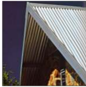
Figure 8.69: Use of galvanised corrugated steel sheeting for the roof.
