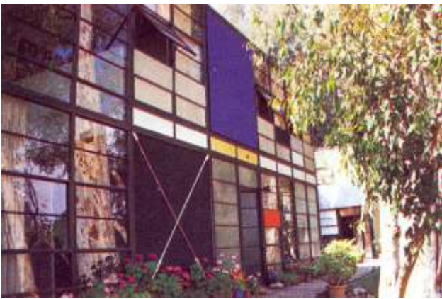
Figure 8.32: Eames House - Charles and Ray Eames. This was an aesthetic based on technology. This building was one of the first 'patter-book' buildings, using components that could be ordered from catalogues.
