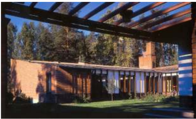
Figure 8.16: Interior view of the courtyard of Säynätsalo Town Hall, Jyväskylä, Finland - Alvar Aalto Aalto's use of brick and timber has a cultural reference in that these materials are widely used in Finland. The massing quality of the brick produces strong and bold forms.
