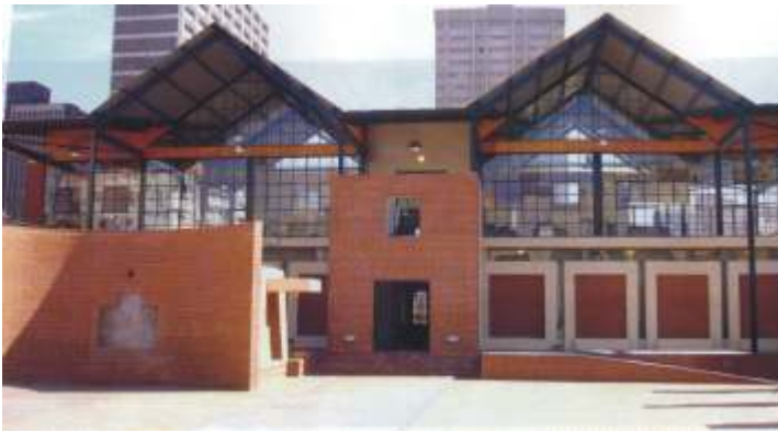
Figure 6.59: Drill Hall, Johannesburg - Michael Hart Architects, Urban Designers cc The transformation of the hall is an example of a responsible design intervention on a historical site. Elements from the original building was reintroduced, such as the form and the use of red brick, while the transformation of the hall is represented by the use of new materials such as off-shutter concrete and full-height glazing.
