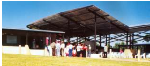
Figure 6.66: Izingolweni clinic and community center, The farm 'Eden', Kwazulu Natal - Llew Bryan Architects and Ashworth Burke Partnership.
