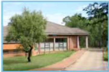
Figure 6.29: Training auditorium Weskoppies is a training hospital for the University of Pretoria. The auditorium is mainly used by for the students for lectures.
