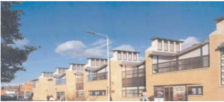
Figure 6.13: Ventilation chimneys link each room to a low level inlet and a high level outlet
