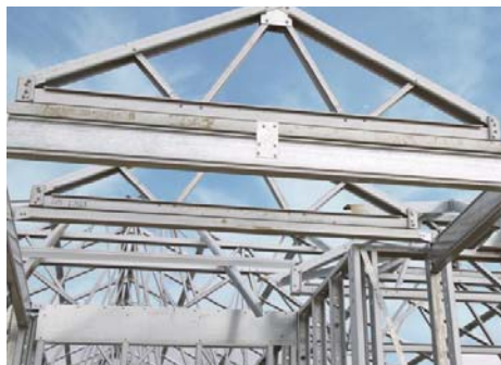
Fig. 7.34: Light gauge steel trusses
