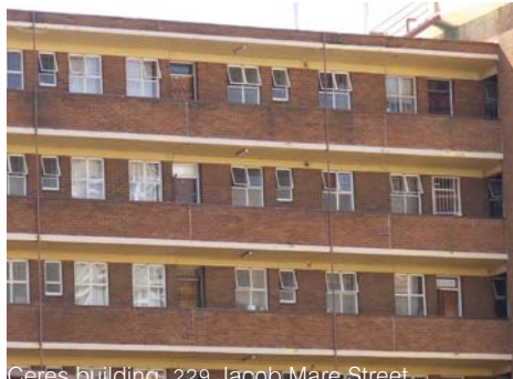
Ceres building, 229 Jacob Mare Street Fig. 5.7: Masonry and exposed structure
