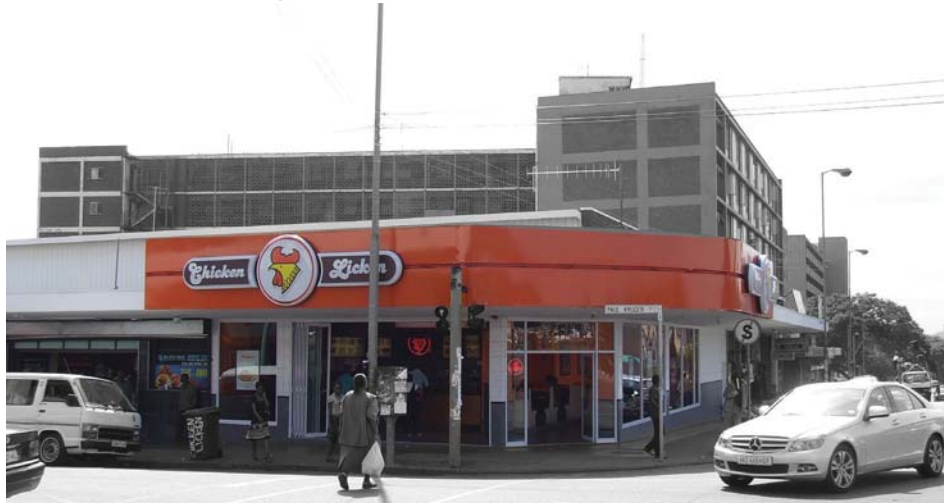
Fig. 1.8: Existing building on site
