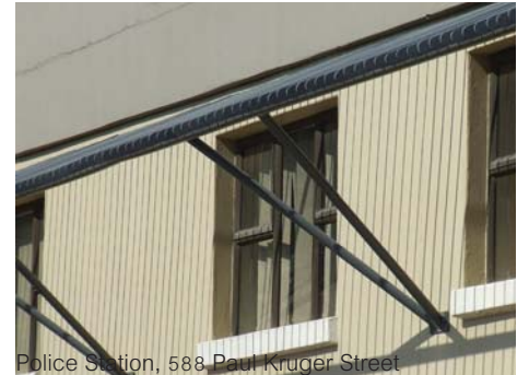
Police Station, 588 Paul Kruger Street Fig. 5.16: Smooth plaster finish and steel shading
