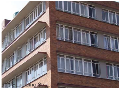
179 Scheiding Street Fig. 5.8: Masonry and steel window frames
