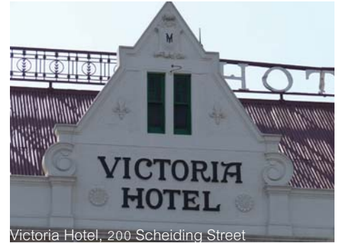
Victoria Hotel, 200 Scheiding Street Fig. 5.15: Decorative plaster finish
