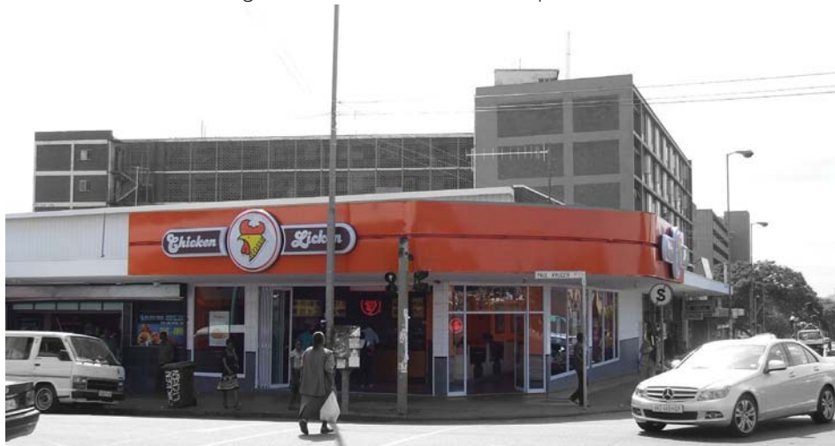
Fig. 1.8: Existing building on site
