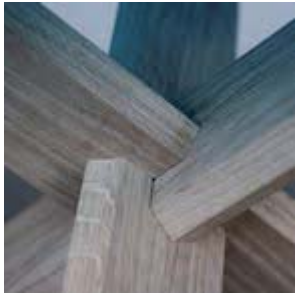
FIGURE 5.21 Cut-out shape joint by ding3000
