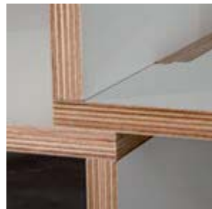
FIGURE 5.18 Slotted lap joint by Norman Hadler
