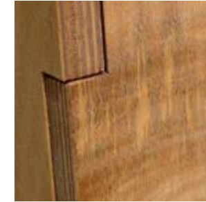
FIGURE 5.13 Barkwadraat magnet joint
