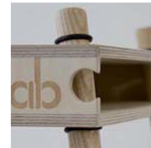
FIGURE 5.14 Poles apart rubber ring joint
