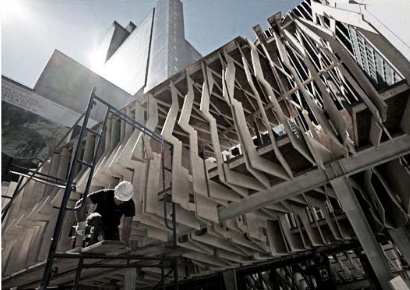
FIGURE 5.44 fin construction: Burst Home (Barnes 2008)
