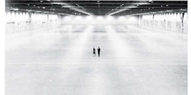
FIGURE 4.5 ExCel exhibition hall (Locker 2011:45)
