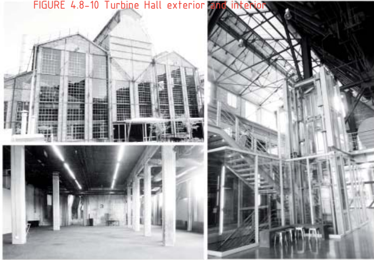
FIGURE 4.8-10 Turbine Hall exterior and interior
