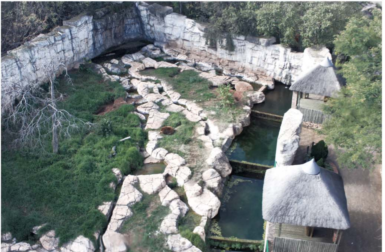
IMG 165: Renovation to Existing Bear Enclosure, from the NZG archives. June 1998 (Photograph by Author, 2011)
