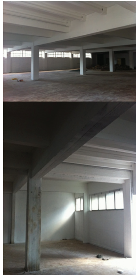
Figure 2.9: Interior of vacant building (Author, 2011).
