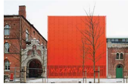
Fig. 58: Public street facade (Lindman, 2010).
