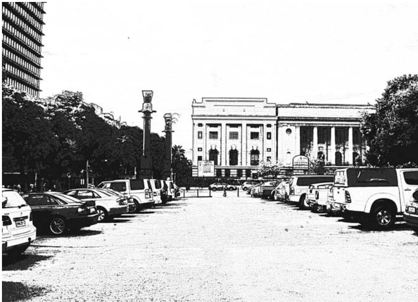
Fig. 36: View of poor edge condition along Visagie Street (Author, 2011).
