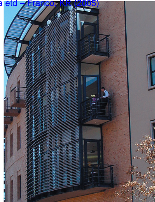
figure 5.20_horizontal aluminium louvres on eastern facade
