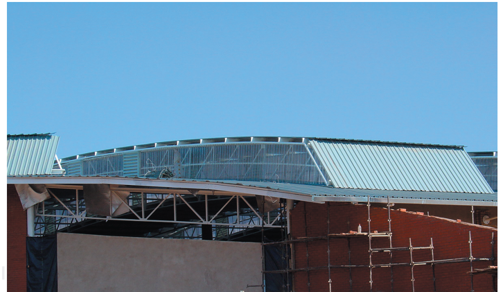
figure 5.22_example of monitor lighting
