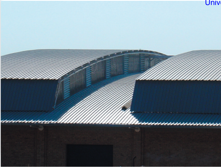
figure 5.23_roof monitors for natural lighting and ventilation
