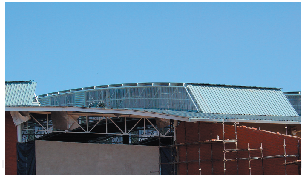
figure 5.22_example of monitor lighting
