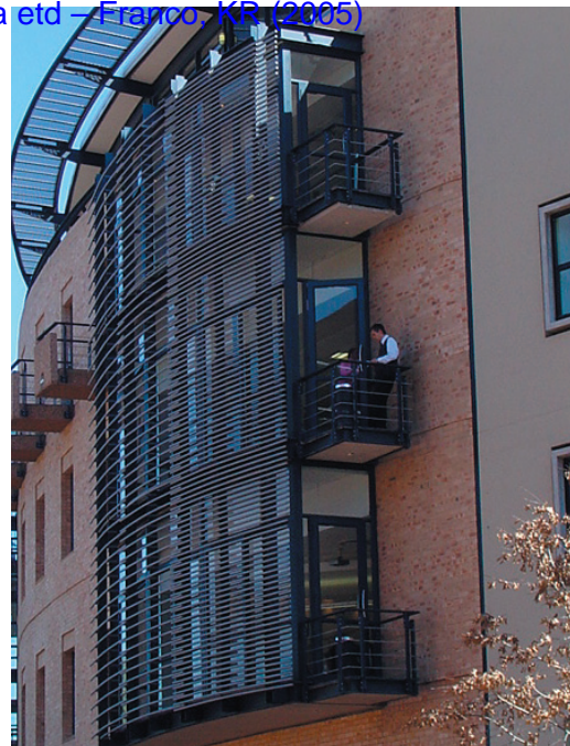
figure 5.20_horizontal aluminium louvres on eastern facade
