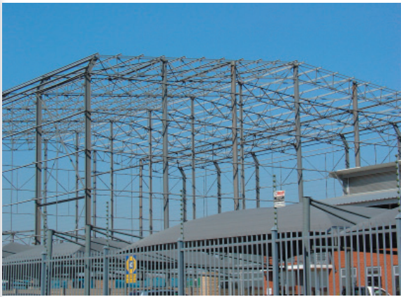
figure 5.03_ steel frame construction
