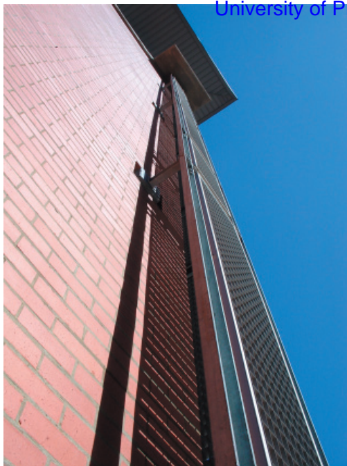
figure 5.19_'mentis' grid sun shading example
