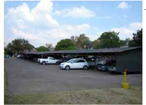
PARKING AREA - BASEMENT PARKING WITH FOUR STOREY BUILDINGS IN FRONT PUBLIC SPACE
