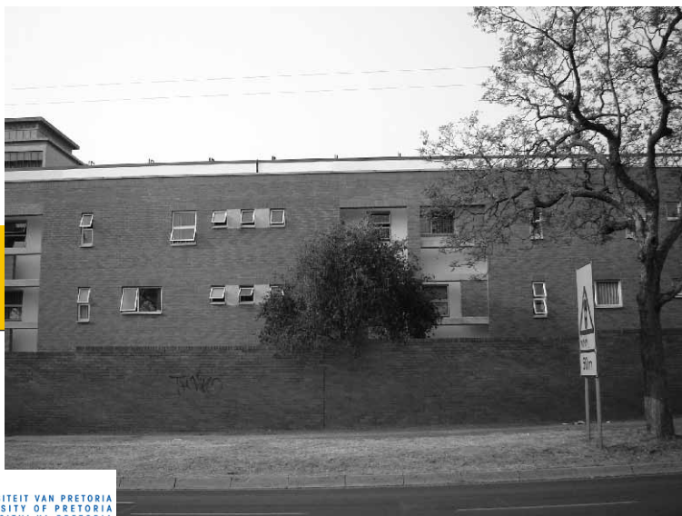
FIG 6-33: EXISTING FACADE OF THE NERINA EXTENTION
