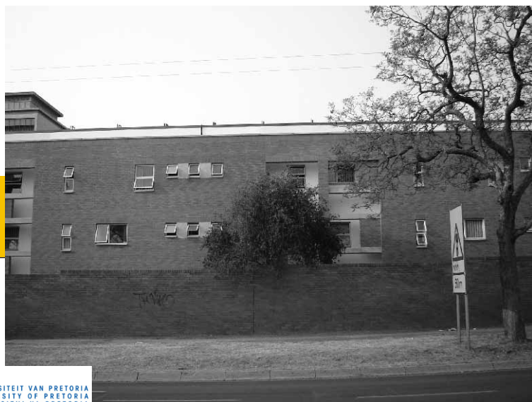
FIG 6-33: EXISTING FACADE OF THE NERINA EXTENTION
